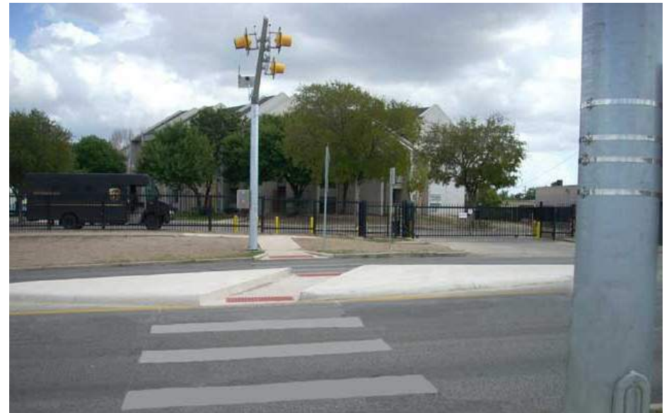
Above: Mid-Block Path Crossing with Refuge Island.
